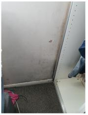
Visible mould contamination to the entire external wall, most of the contamination appears to be located behind the wardrobe which is situated along the partition wall dividing bedroom and kitchen. Back of the wardrobe is also showing signs of mould contamination.
