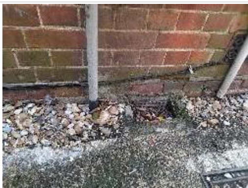
Visible slate dpc just above French gully. Airbrick partially blocked by gravel/debris
