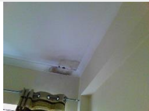
Photo of water damaged area of bedroom ceiling, coving and upper wall.
