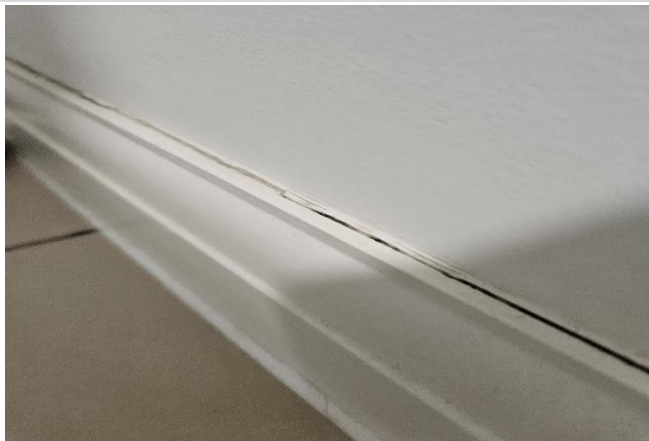
Debonding of the skirting board from the wall behind
