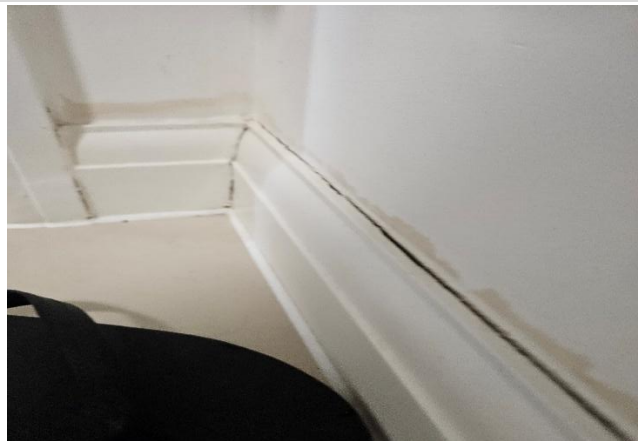
Swelling & debonding of the skirting board, staining of the lower wall`
