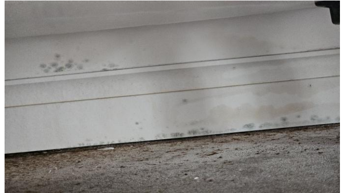
Fungal colonisation along skirting board and lower wall
