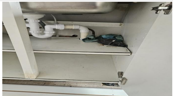
Widespread swelling and staining of the sink cupboard
