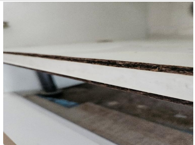
Swollen particleboard shelf with visible edge delamination indicative of prolonged water exposure.
