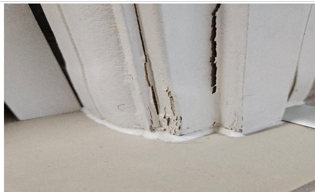
Swelling and cracking of the door frame and architrave
