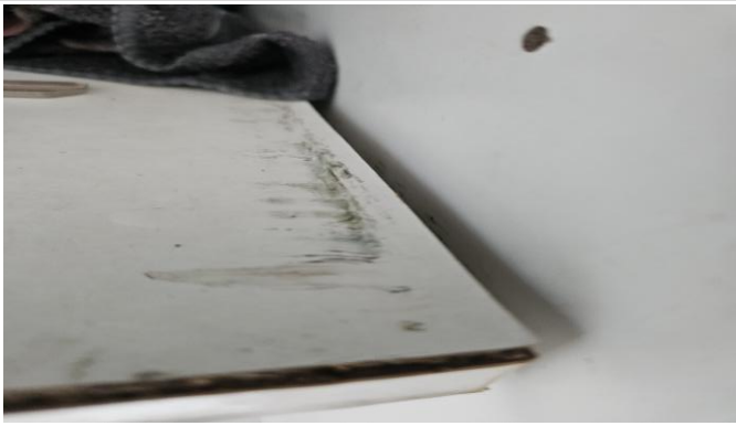
Swelling and mould contamination on the surface of the shelf
