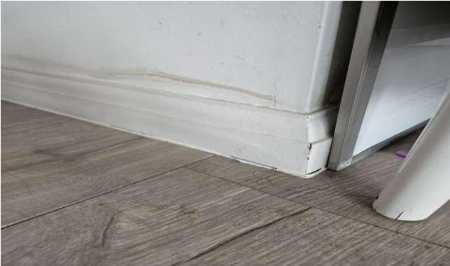
Brown moisture staining to lower wall, swelling of the skirting boards.
