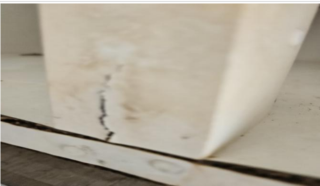
Vertical cracking and edge swelling of internal panel
