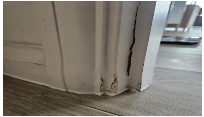
Swelling, splitting of the door frame and architrave, peeling of paint
